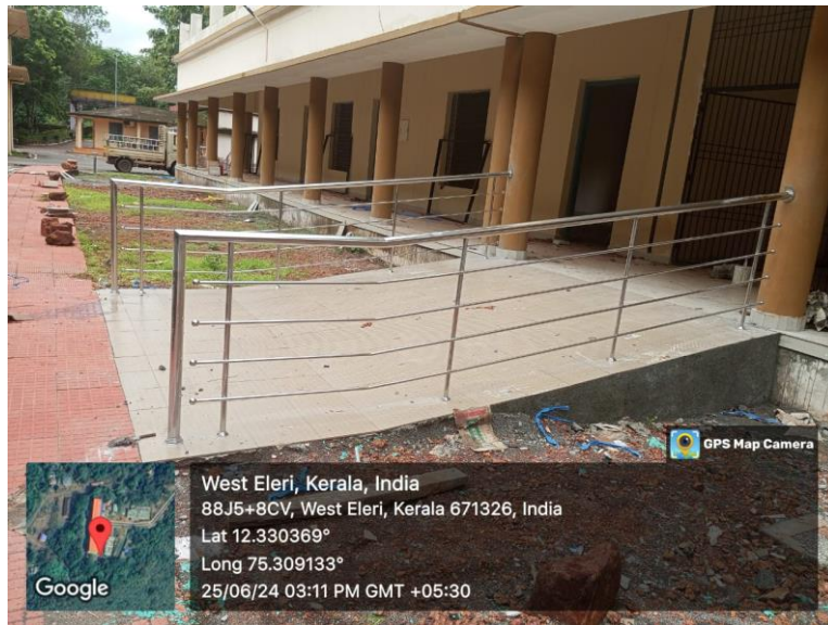
Ramp in the Economics PG Block
