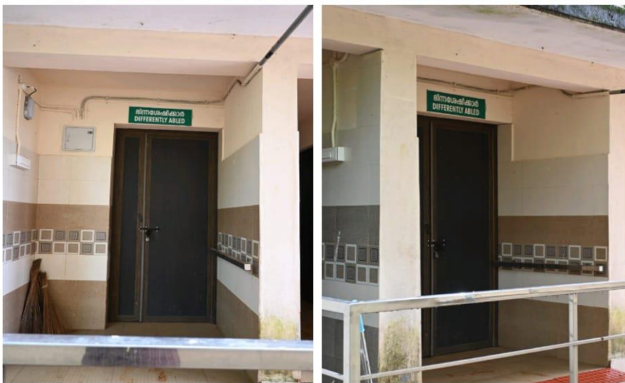
Toilets equipped with Ramp for the Differently Abled Students
