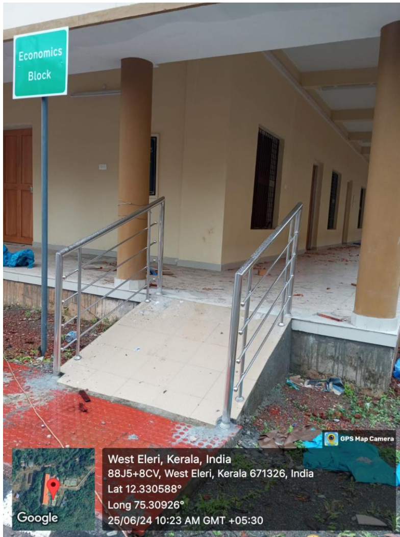
Ramp in the Economics PG Block
